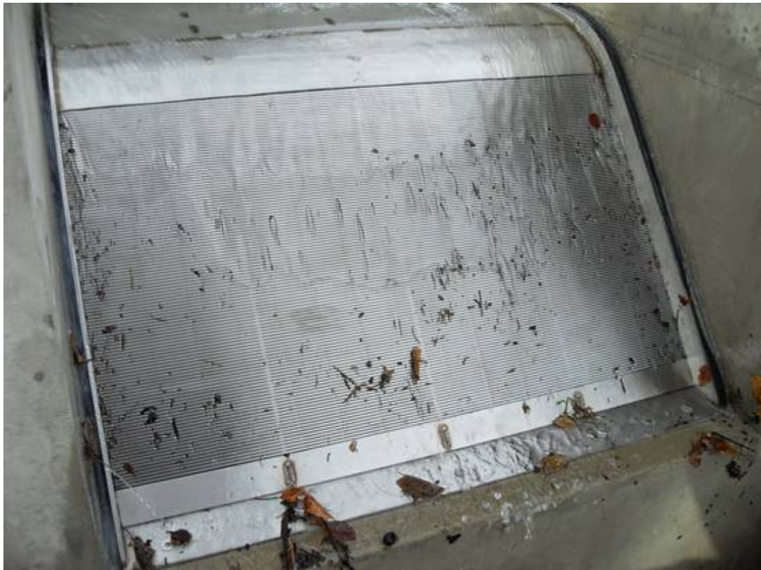
Figure 1 - WRE wedge wire screen
