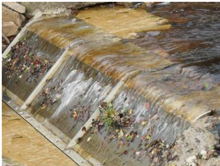
Figure 5 - Wedge wire screens self clean most debris, and are tolerant to partial blinding
